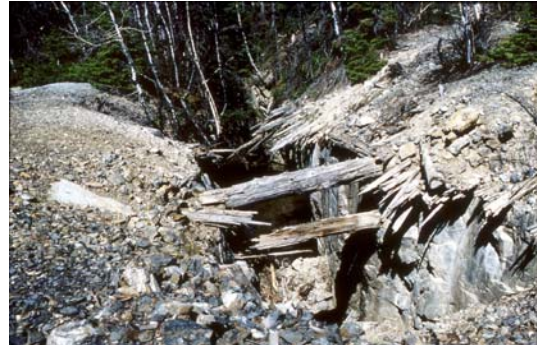
Old copper mine with collapsed rotten log cover
