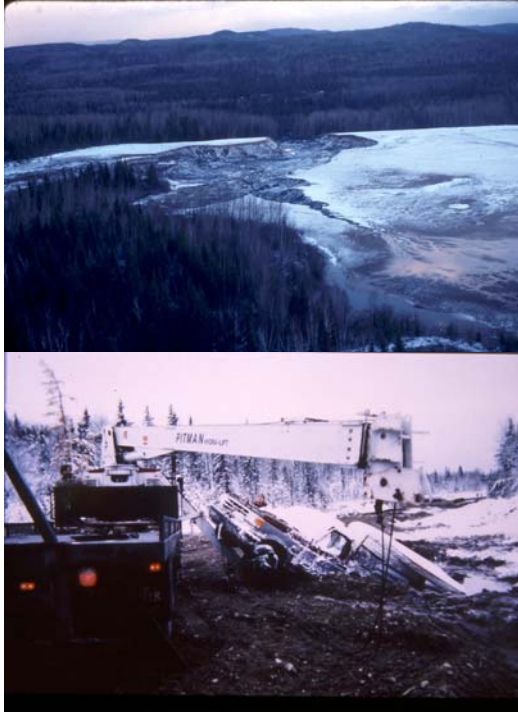
Scar from tailings run-off and pick-up truck entrapped in the tailings
