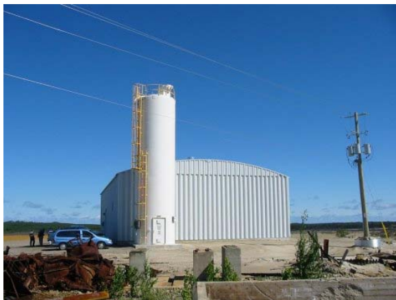
New treatment plant at Kam Kotia site
