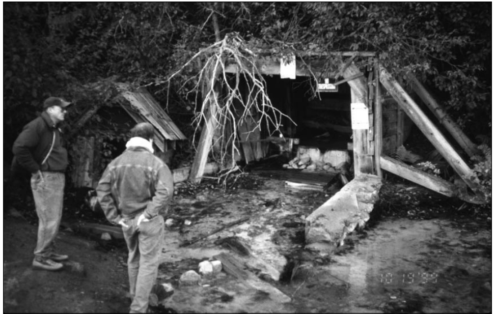
Figure 2. Mine portals and adits such as this one at the Holden Mine can be dangerous physical hazards and sources of water pollution when acid mine drainage is generated and metals are transported to surface or ground water.
