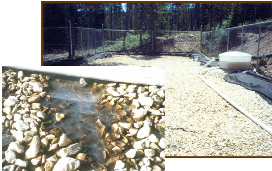
Figure 6. Aerobic bioreactor with manganese deposits.
